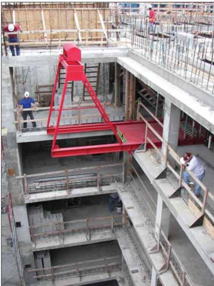
As an accessory, Kern Baxter's LTD4000 load lifting transfer deck operates independently, delivering materials into the building, and freeing the crane to perform more critical duties on a high-rise jobsite.
